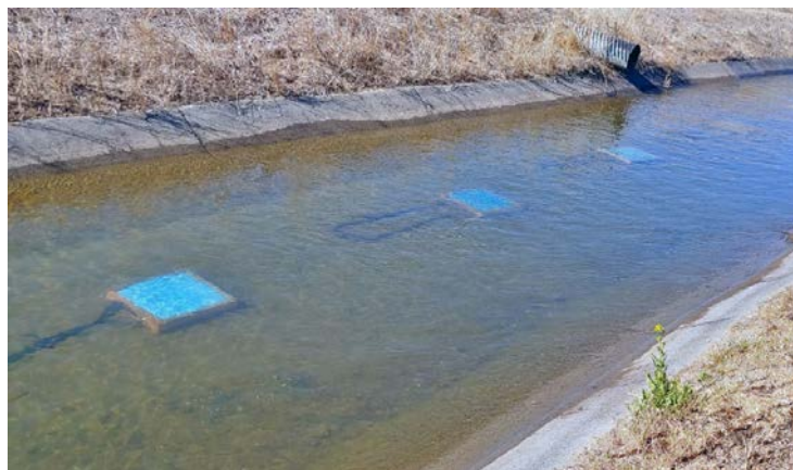
Coated concrete panels in canal during testing.
