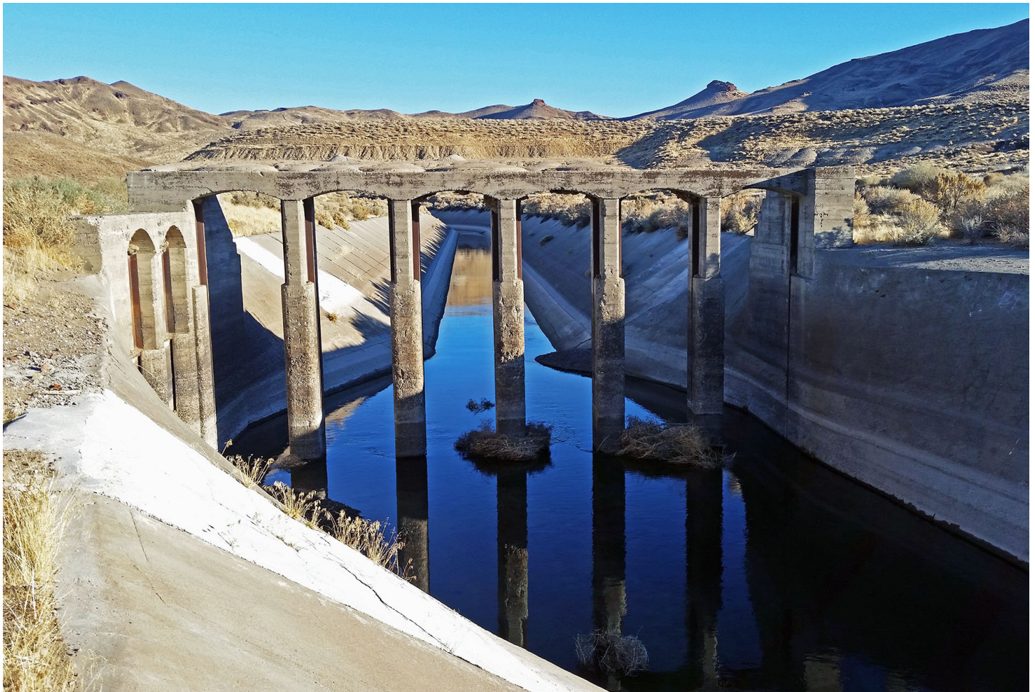
Truckee Canal structure - Photo credit Ramon Naranjo, USGS.
